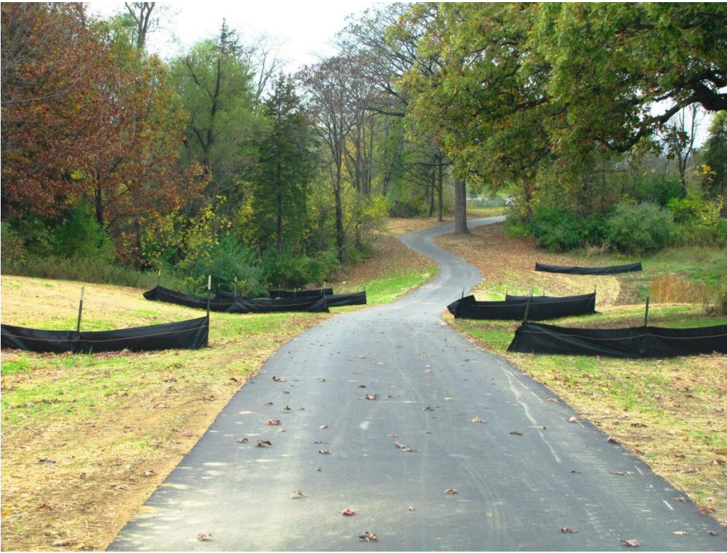
Completed trail – Photo taken October, 2011.
